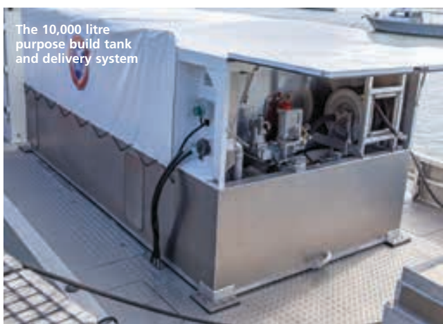
Tidy machinery spaces below
